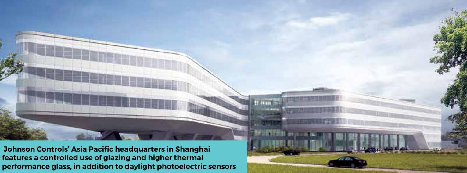
Johnson Controls' Asia Pacific headquarters in Shanghai features a controlled use of glazing and higher thermal performance glass, in addition to daylight photoelectric sensors
