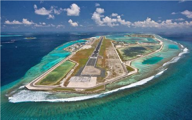
Ibrahim Nasir International Airport
